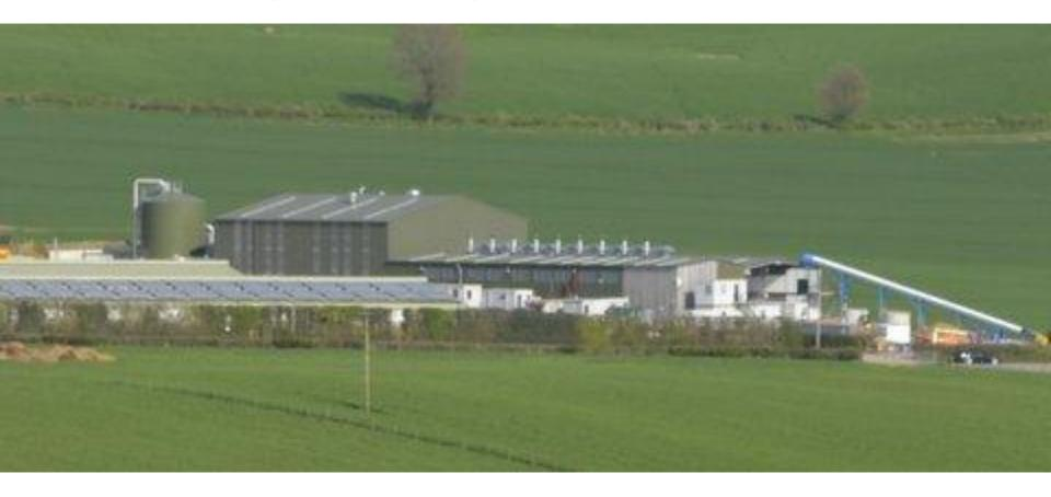
With exception of delivering the gasifier (Eco-Cycle/Torftech) Dordtech provided: Engineering and construction; all piping and electrical connections; Over-All control technology of all major components
