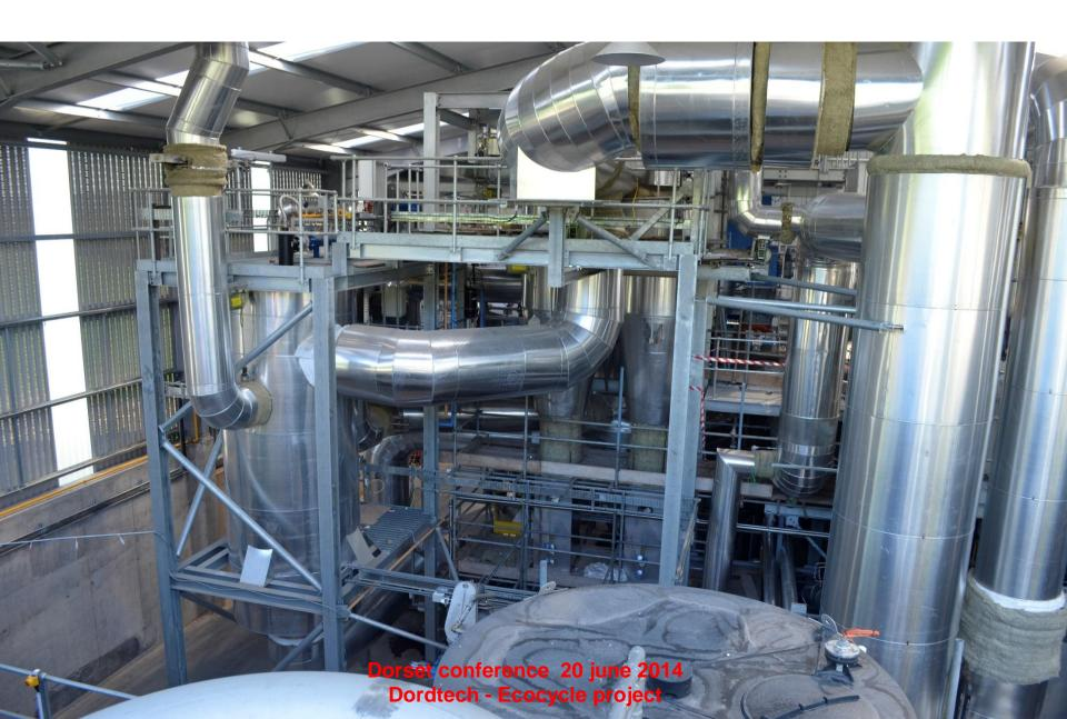
WESP = Wet ElectroStatic Precipitator for removal of solid particles and liquid droplets from the gas stream
