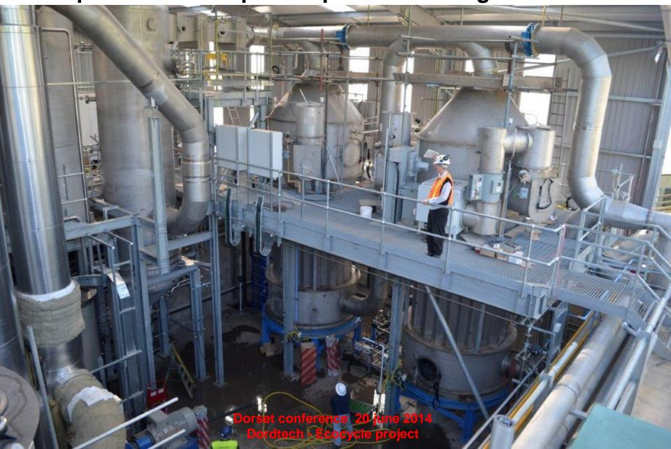
Heat from the CHP units is used for the absorption chiller to produce water of 6°C to cool the syngas
