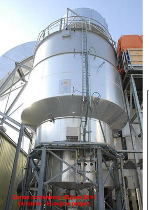
Woodchips are gasified In the Torftech gasifier at aproximately 700°C with minimum O2.
